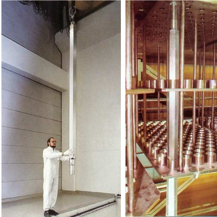
Fig. 4.3.9 Fresh nuclear fuel storage in Finnish nuclear power plant Loviisa. [Imatran Voima Oy: Loviisa Power Plant]
