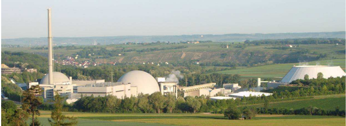
Fig. 4.3.36 View of Neckarwesheim power plant (Germany) with a hybrid cooling tower in unit II (unit I is cooled in open cycle from the river Neckar with auxiliary fan cooling towers)
