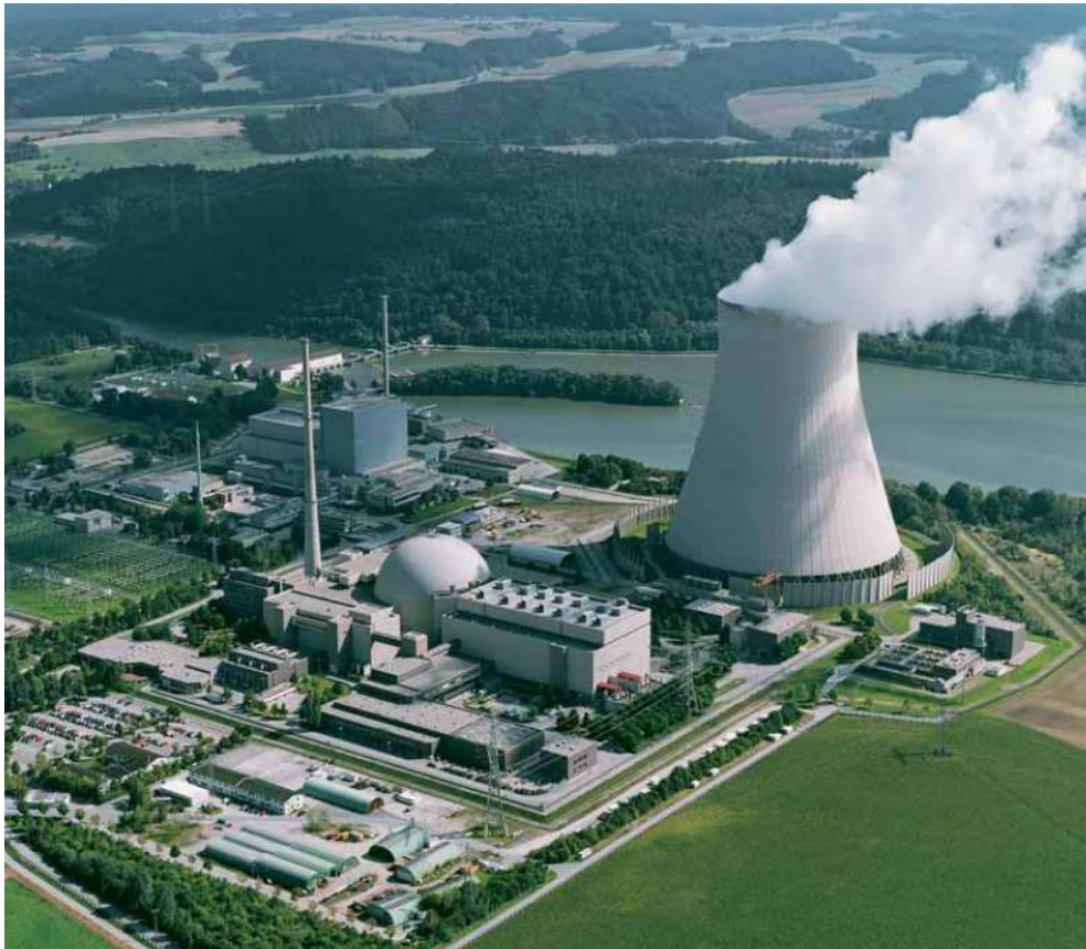
Fig. 4.3.31 Nuclear power plant Isar II (Germany) with wet natural draught cooling tower.
