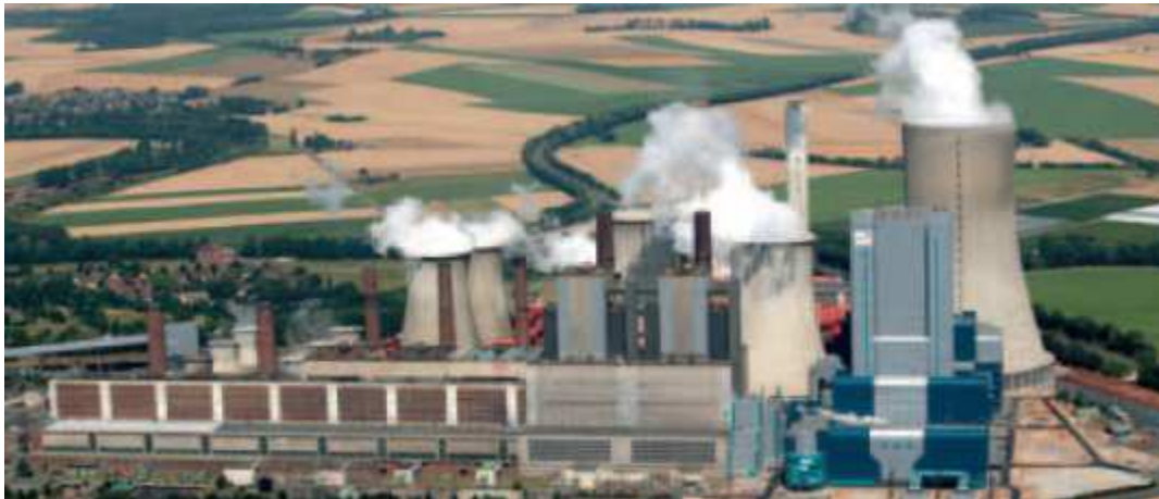
Fig. 4.3.33 Niederaussem power plant (Germany) with the tallest wet natural draught cooling tower in the world (200 m)
