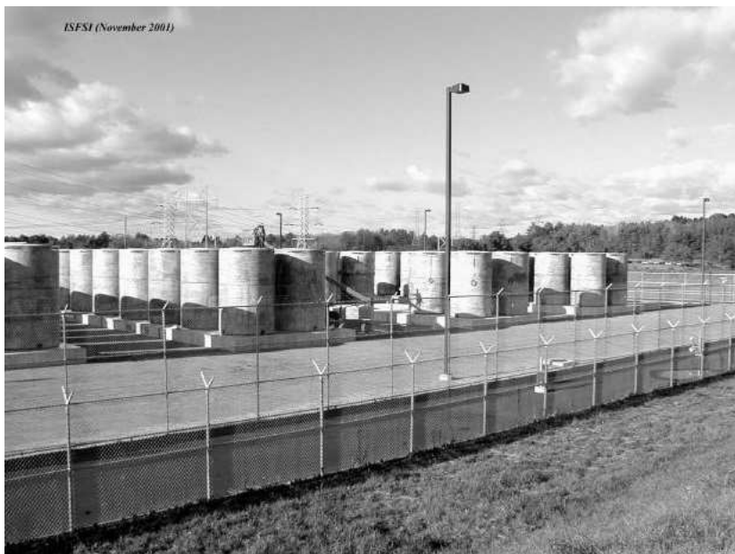
Figure 3.1.3. Containers with spent fuel left at the former Maine Yankee site.
